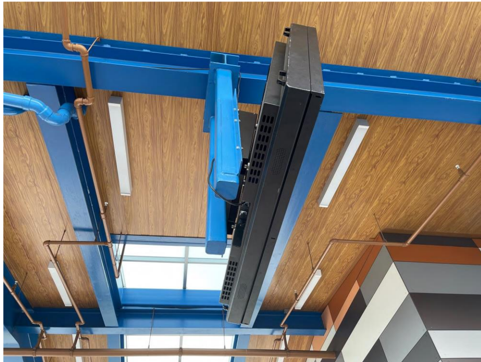
Figure 4: NANO V 55" Outdoor Single-Sided Real-Time Passenger Information Digital Sign with Ceiling Mount in Lauderhill Bus Bay – Bottom View
