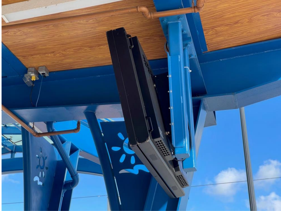
Figure 3: NANO V 55" Outdoor Single-Sided Real-Time Passenger Information Digital Sign with Ceiling Mount in Lauderhill Bus Bay – Side View
