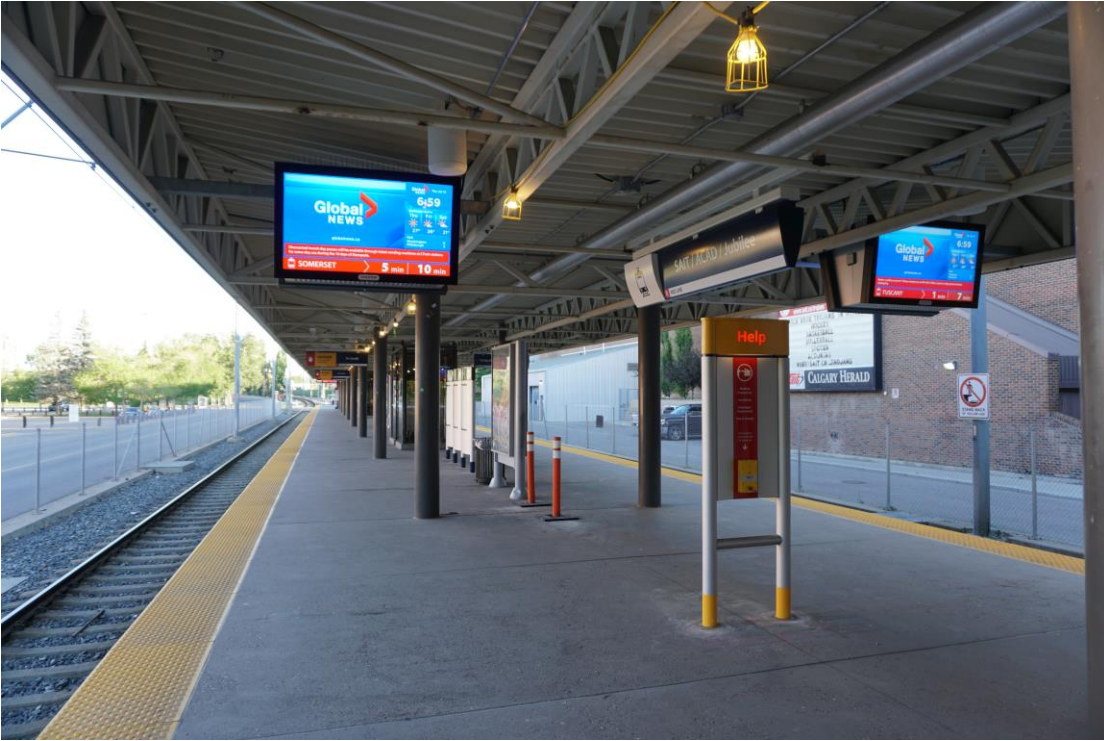
Figure 6: NANOV 55" Single-Sided Passenger Information Display Signs (PIDS) at SAIT/ACAD/Jubilee Red Line CTrain Station in Calgary, Alberta
