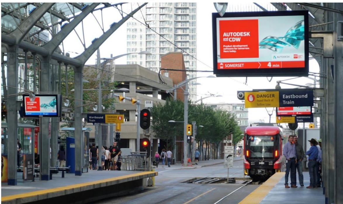
Figure 2: NANOV 55" Single-Sided Passenger Information Display Signs (PIDS) at CTrain Station in Downtown Calgary
