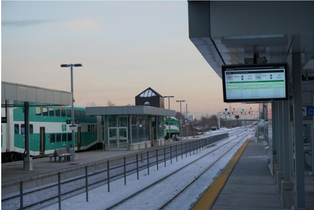
Figure 5: NANOV 46" Outdoor Real-Time Single-Sided Transit Sign featuring ceiling mount at GO Transit & UP Express Weston Station in Toronto, Ontario.
