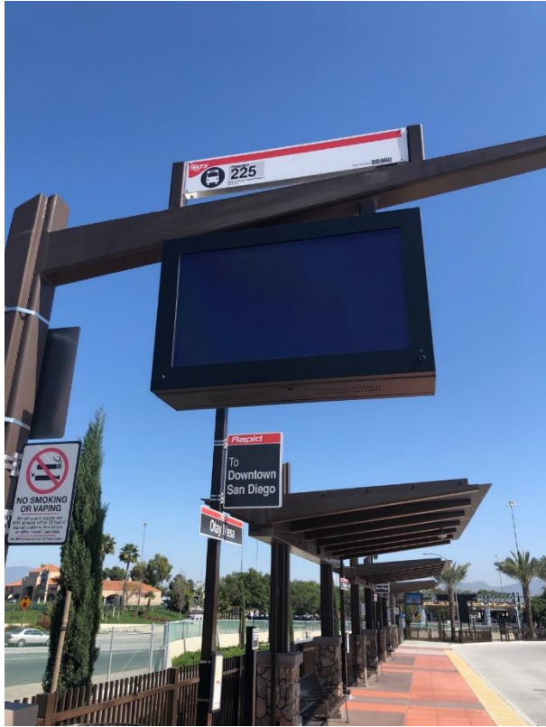
Figure 7: NANOV 46" Double-Sided Real Time Variable Message Sign (VMS) in San Diego Rapid Bus Service Station
