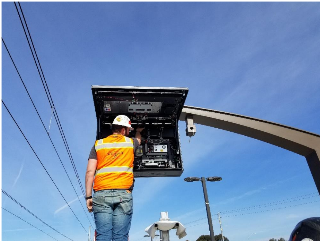
Figure 6: Installation of NANO V 46" Double-Sided Real Time VMS in San Diego Rapid Bus Service Station featuring easy-open maintenance access doors
