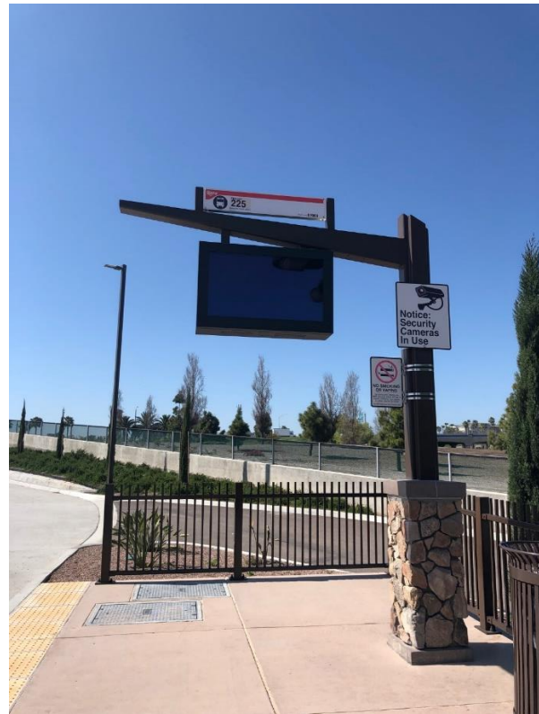
Figure 8: NANOV 46" Double-Sided Real Time Variable Message Sign (VMS) in San Diego Rapid Bus Service Station
