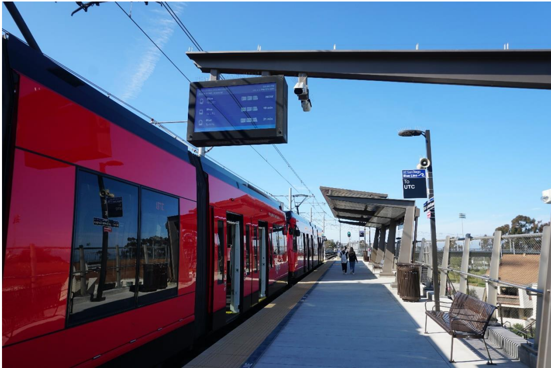
Figure 3: NANOV 46" Double-Sided Real Time Variable Message Sign (VMS) in San Diego Blue Line Station
