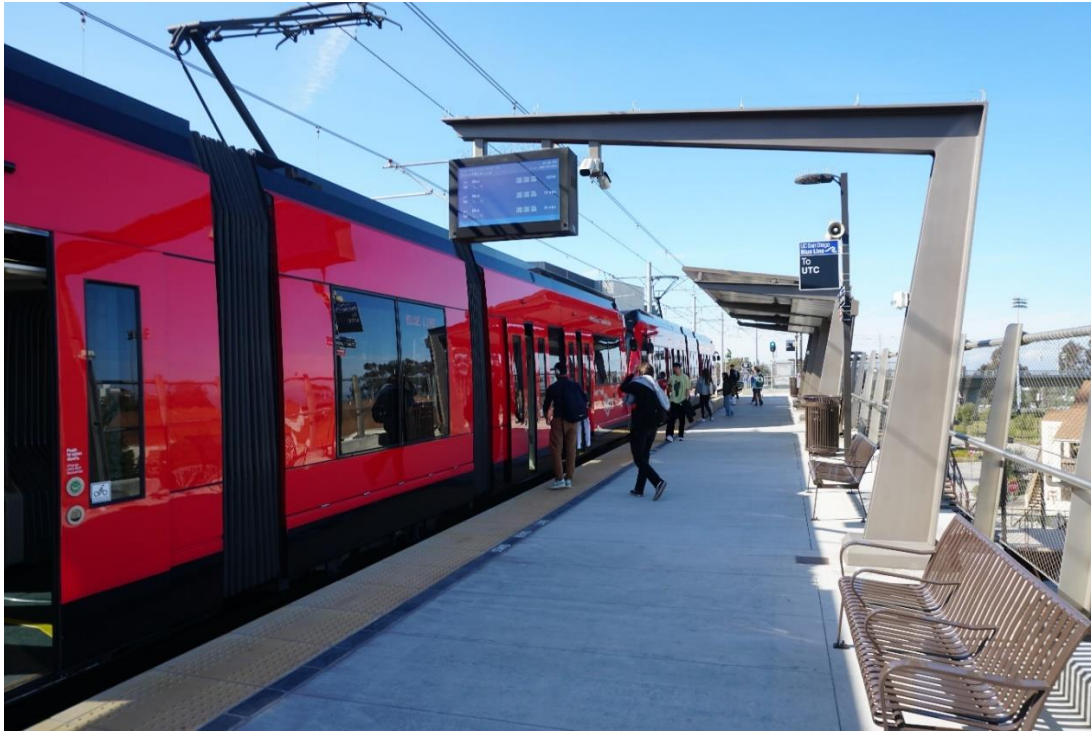
Figure 1: NANOV 46" Double-Sided Real Time Variable Message Sign (VMS) in San Diego Blue Line Station
